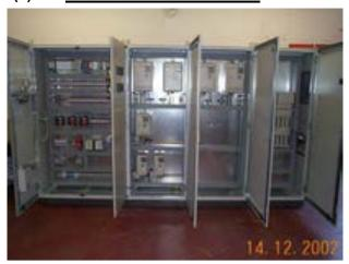
The instruments and controls will be mounted in a completely enclosed, floor mounted pre-wired **Rittal (with steel plinth)** control panel with front access. The control panel will include motor starters, selector switches, fused disconnects, pilot lights, flame safety relays, a fixed purge timer, burner controls, fused branch circuits, a 24 VDC control transformer, a main disconnect switch with a door interlock and a **Rittal** panel air conditioner.
