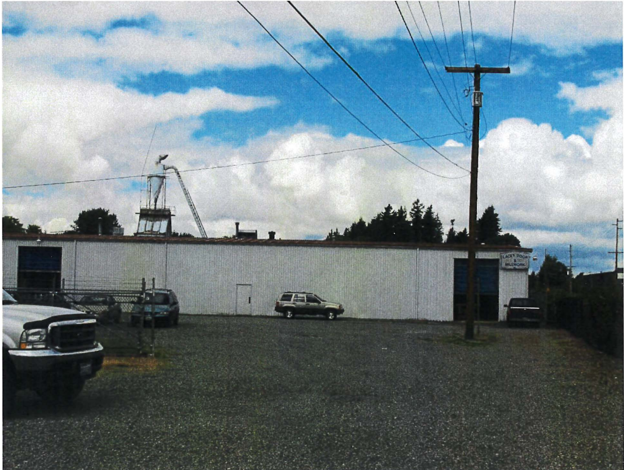
Figure 3.2: Picture of Facility
