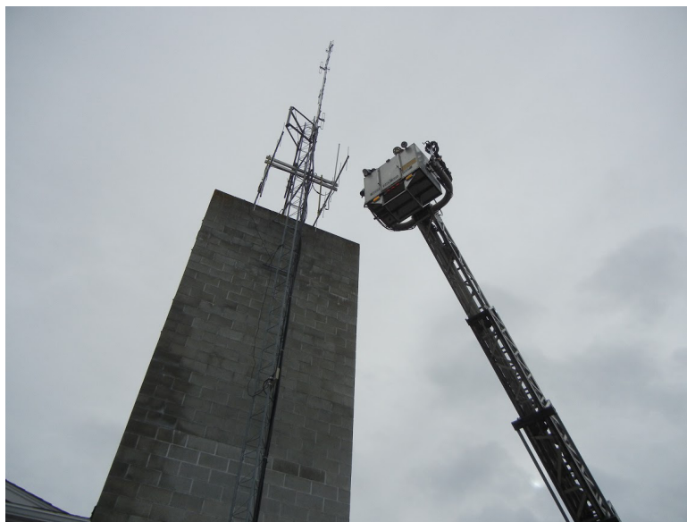
Installing the Sequim monitor on the fire station.
