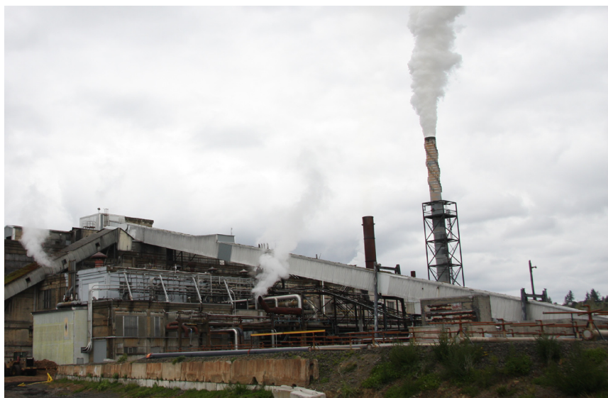
Grays Harbor Paper in Hoquiam is one of the many businesses ORCAA works with to ensure air quality laws are met. As can be seen in this picture, the stacks at the plant frequently emit steam vapor which is allowed.
