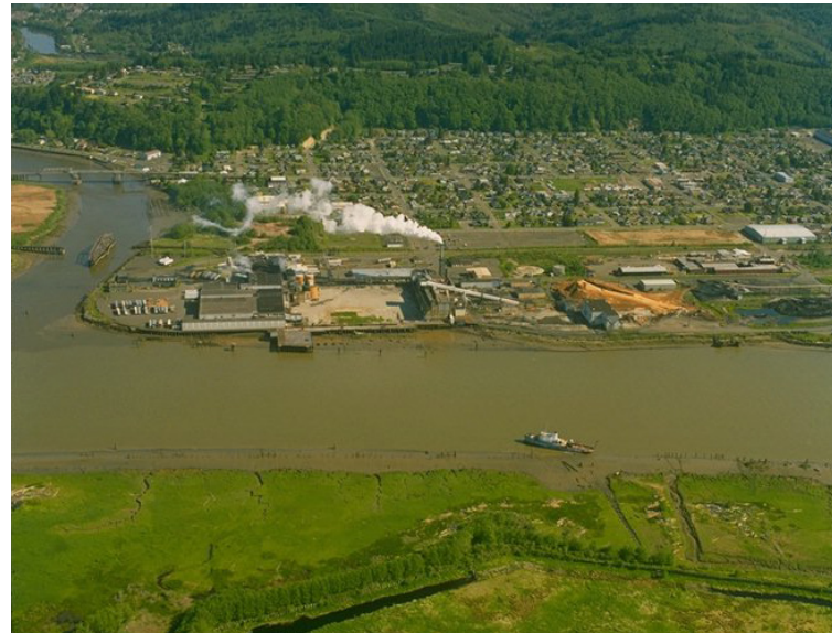
Aerial view of Grays Harbor Paper in Hoquiam.
