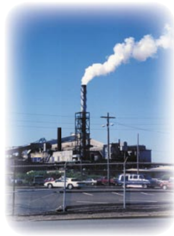
The Engineering section provides technical assistance and regulatory oversight of major sources in ORCAA's jurisdiction.
